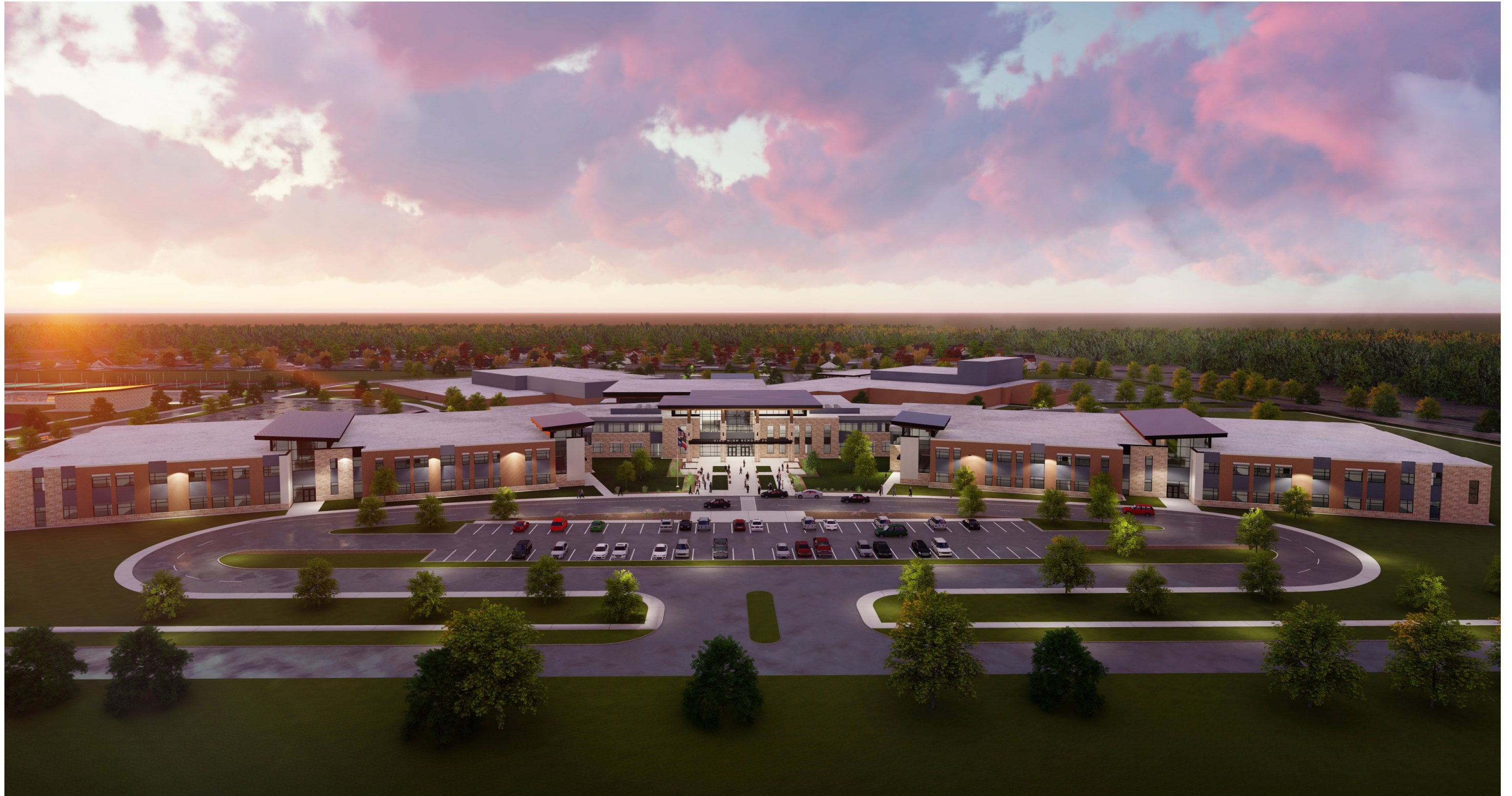
VIEW OF MAIN ENTRY AT DAWN
